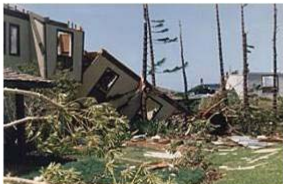
Disasters such as hurricanes can severely impact Hawaii's energy supply and distribution infrastructure.
